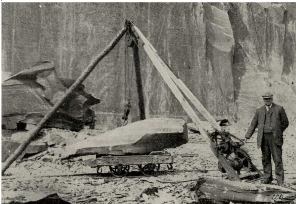
FIG. 3.—SAFETY HAND-WINCH.
