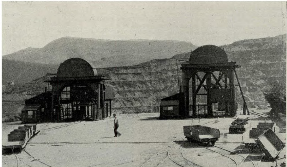
FIG. 2.—WATER-BALANCES AND THE QUARRY IN THE BACK-GROUND.
